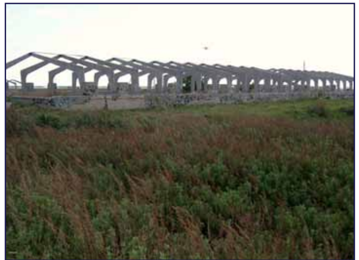
Source Al Scholz – Abandoned dairy barn
